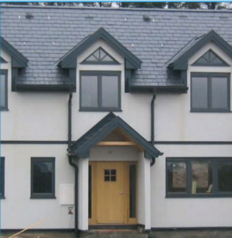
Promat PROMATECT®-B cladding with polymeric render on timber frame house
